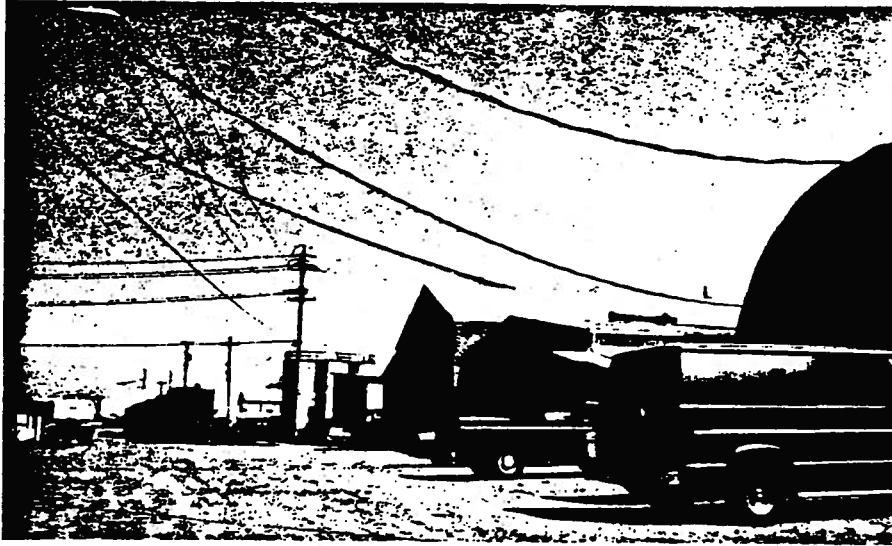
9 Many of the industrial structures along Wills Road (Subarea 1-1) are marginally maintained, the area is devoid of landscaping, and the lack of paved street improvements contributes to haphazard parking practices and poor drainage.
